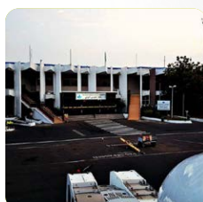
Ambouli International Airport (Djibouti City)
