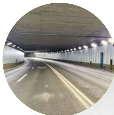
Bonanova Tunnel (Barcelona)
