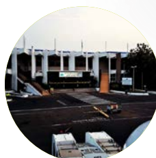
Ambouli International Airport (Djibouti City)
